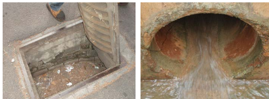
The City manages nearly 28,000 catchbasins and over 1,100 miles of infrastructure, including piped systems.
