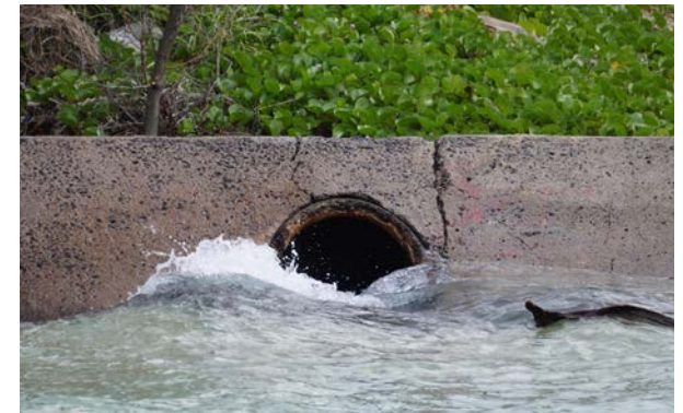
Storm water outlets in low-lying coastal areas become flooded with sea water during King Tide events. High tides are increased by rising sea levels.
