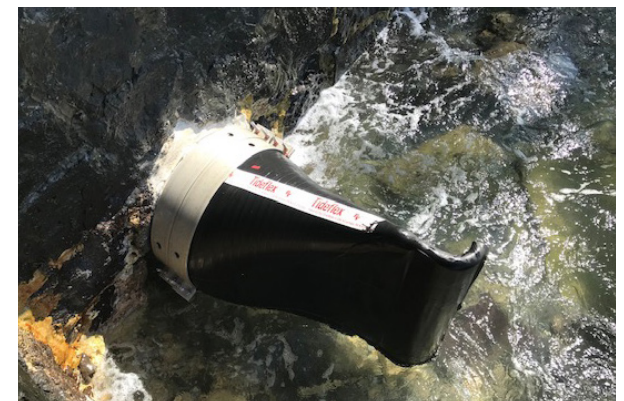
Tideflex duckbill valves are installed at storm water discharge points along the coast to prevent the backflow of seawater into storm flow pipes.
